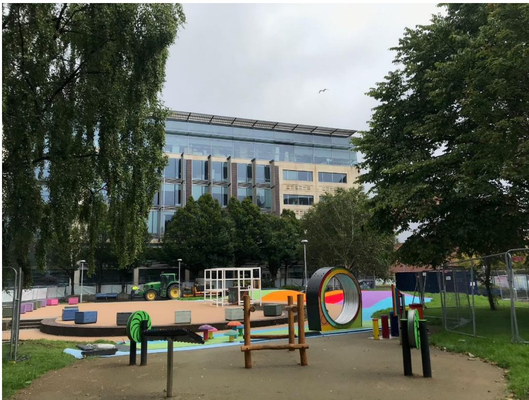
Work in progress (27.07.20).
